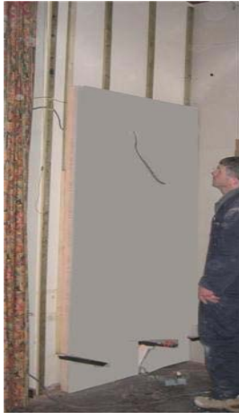
Insulating the walls
